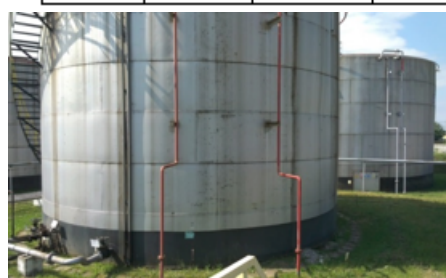
Fig. 4 Crude oil storage tanks which have undergone experimental research
